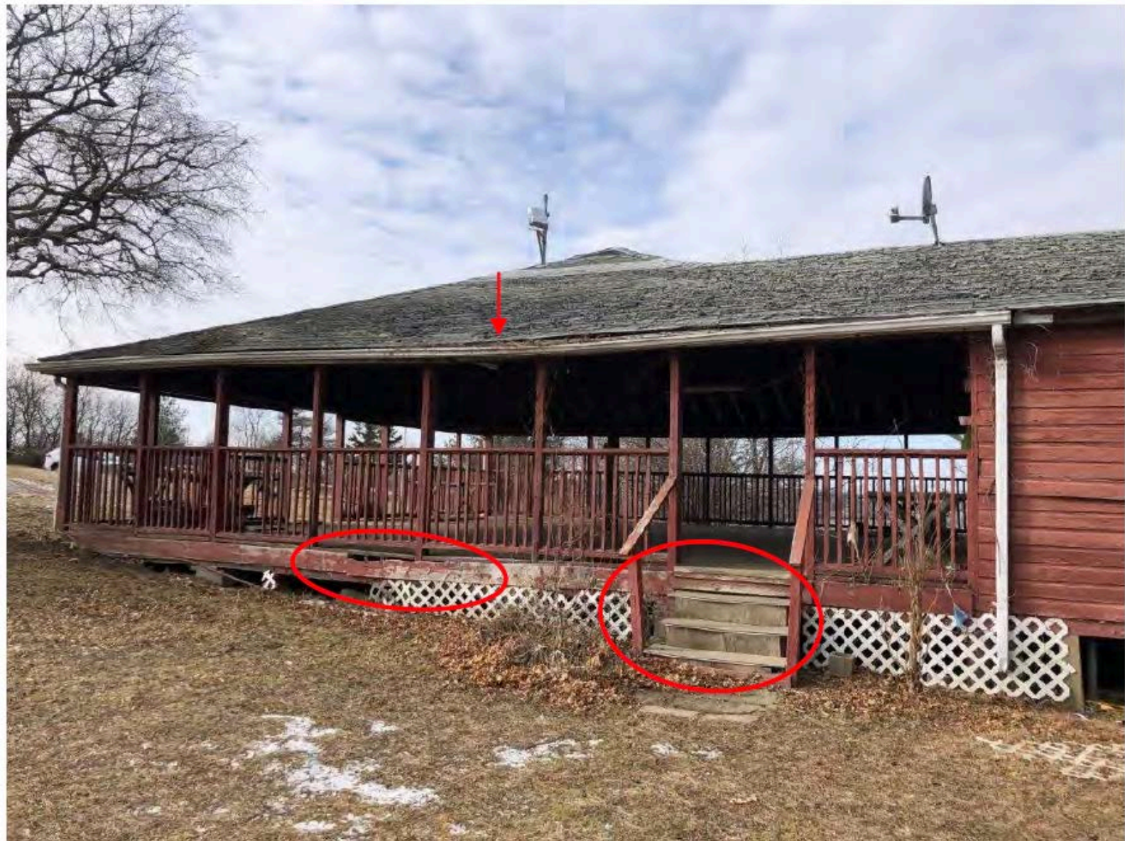
Photo 8: Deteriorated roof, sill and stairs (east elev.)
