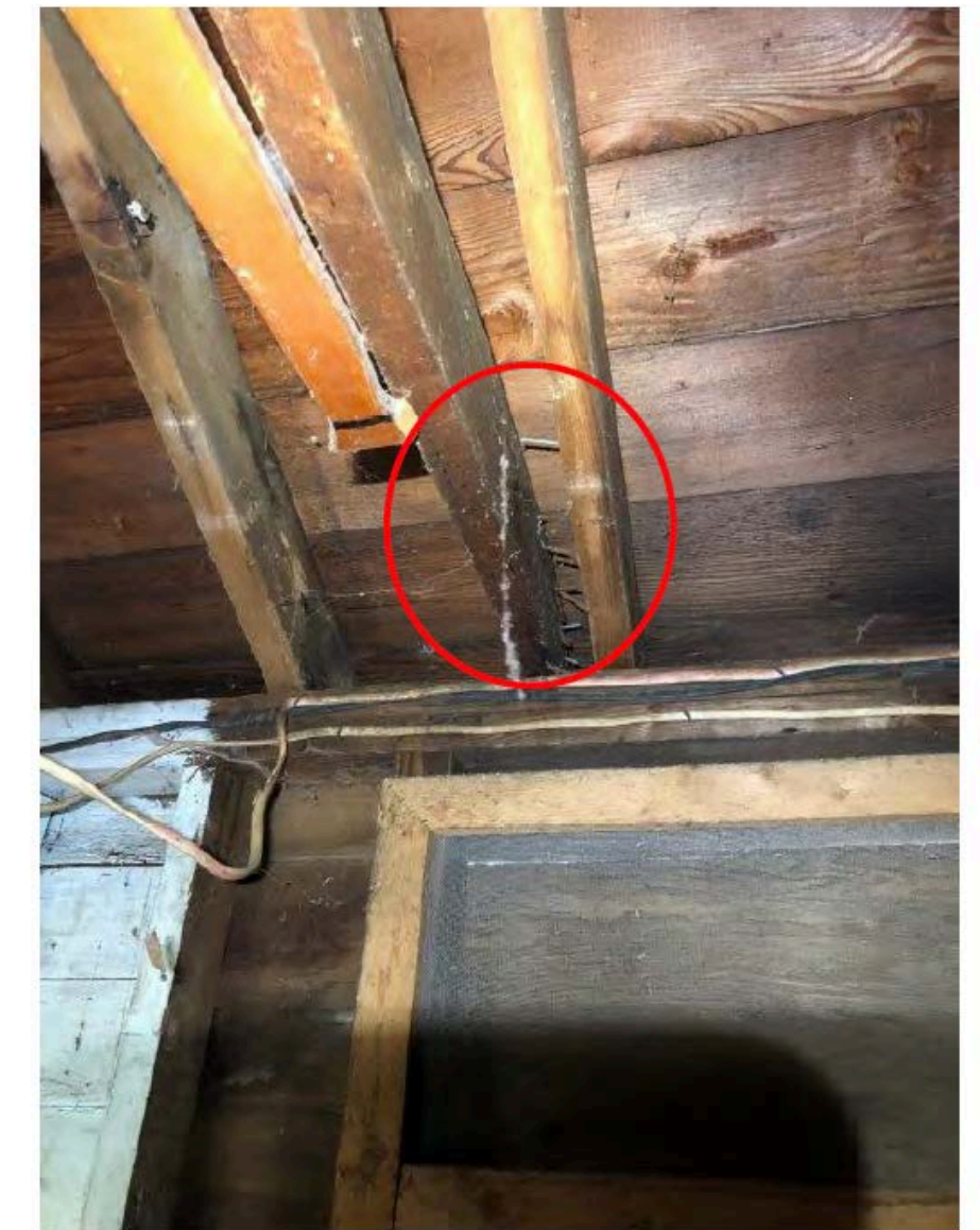
Photo 32: Failed rafter and collar tie connection (facing north)
