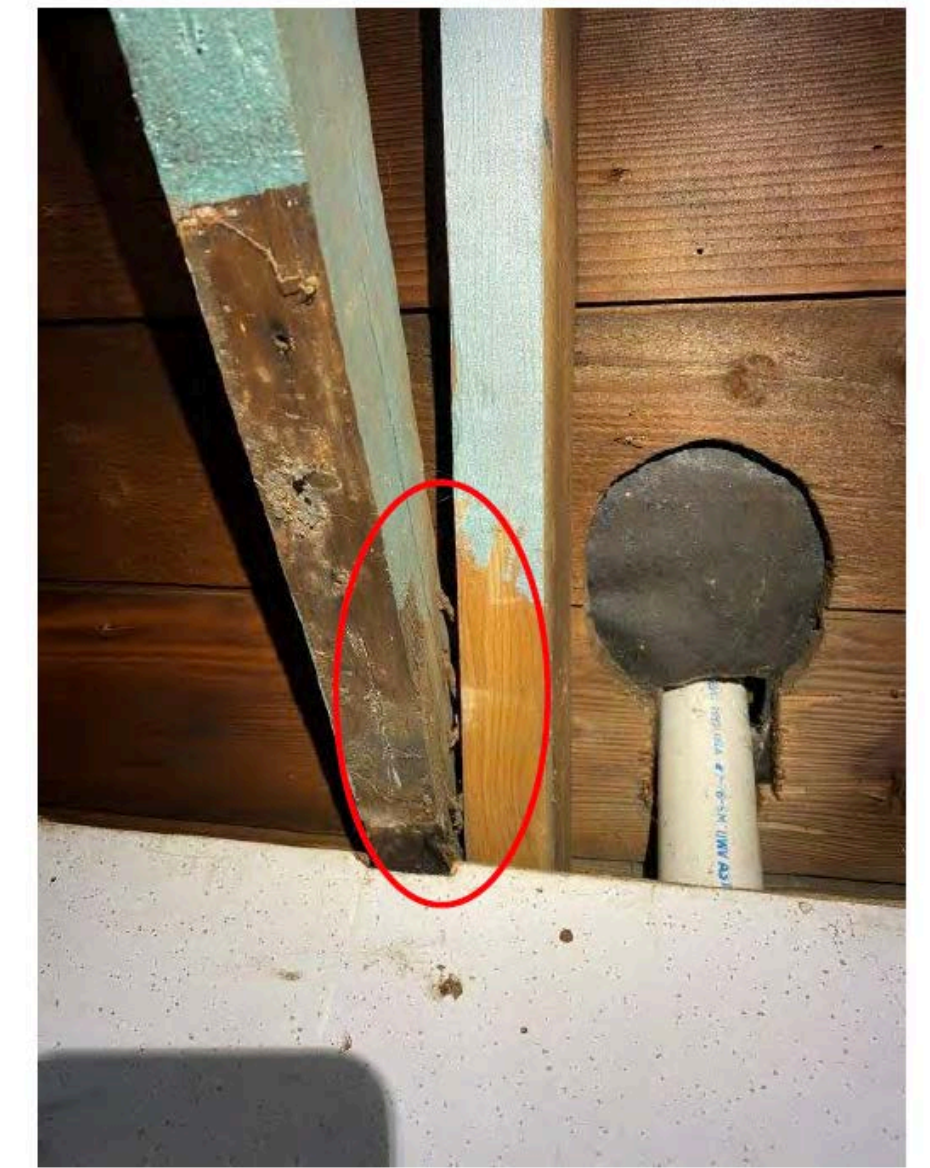
Photo 36: Collar tie and rafter connection failure in Building C
