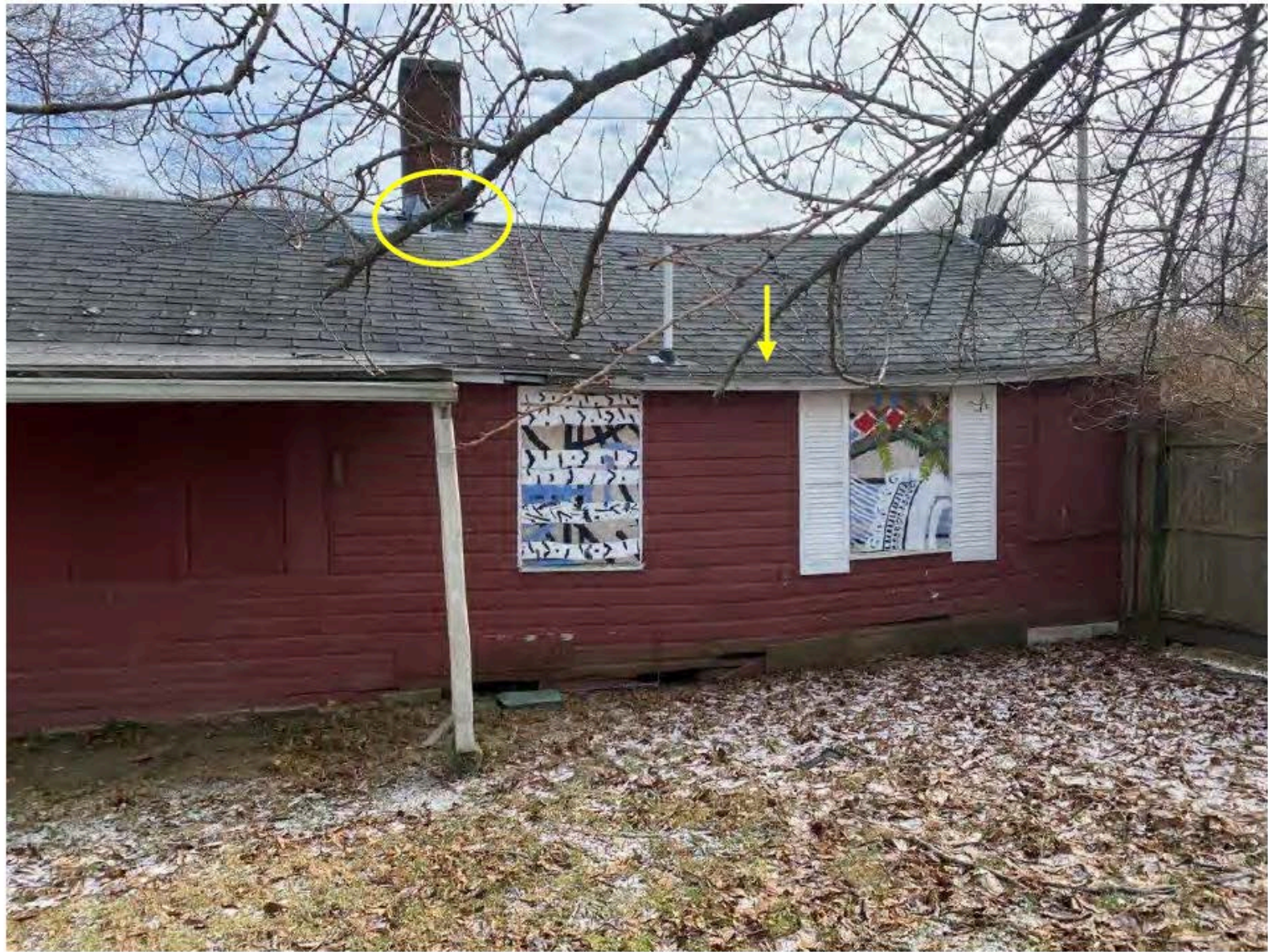
Photo 18: Sagging roof and eroded flashing around chimney (west elev.)
