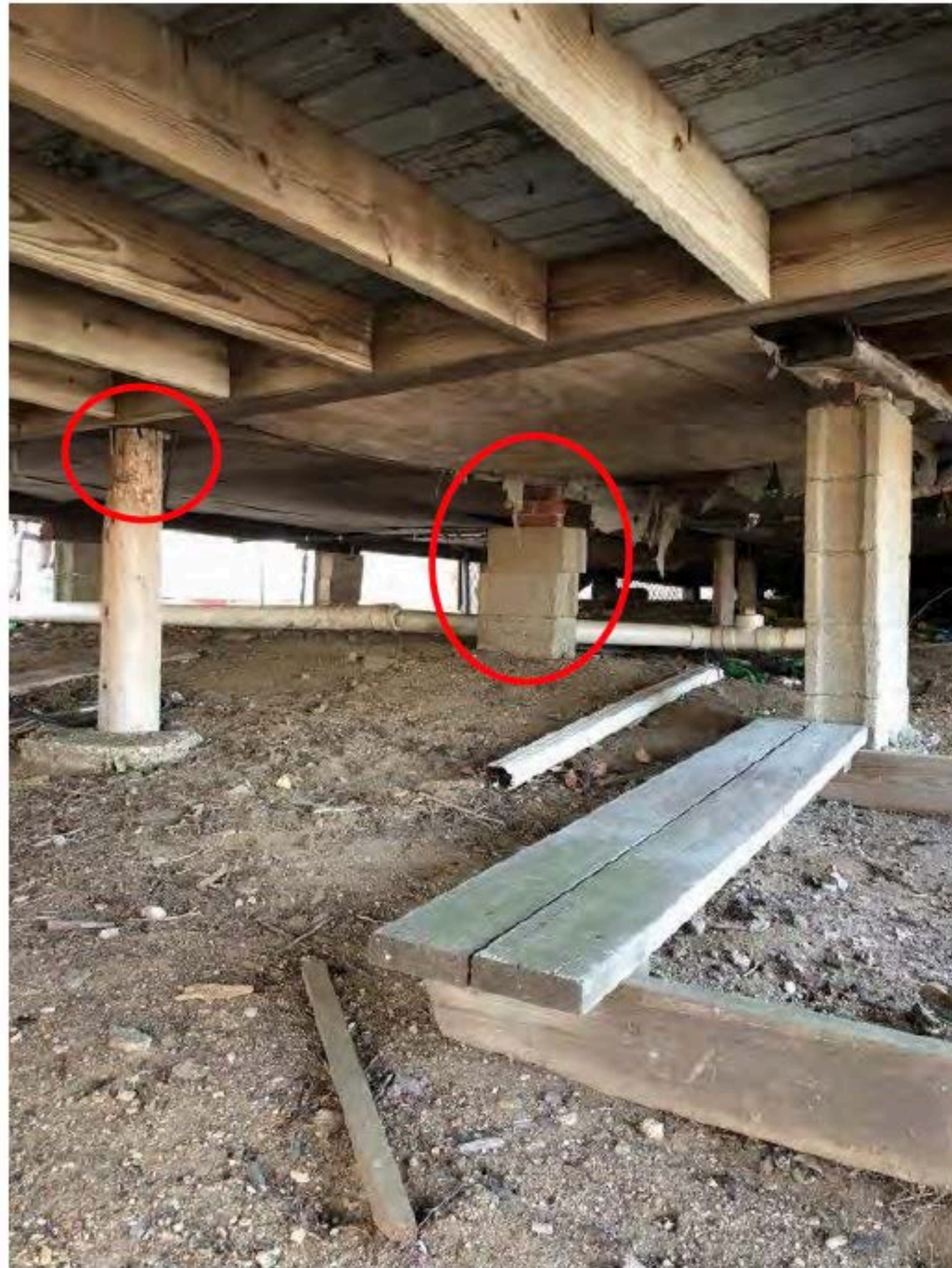
Photo 10: Rotted wood posts and shifted CMU piers
