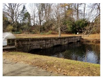
Build up of debris under the Dickson Bridge deck has resulted in spalling, cracking and delamination of the concrete.
