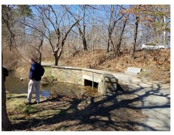
Build up of debris in the culvert at the north end of Sargent Pond has led to failure of the culvert headwall.
