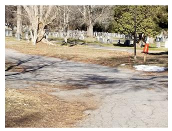
Bituminous pavement throughout the cemetery shows signs of water build up resulting and cracks and failure.
