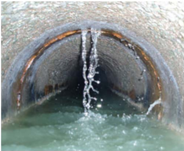
Infiltration into a sanitary sewer
