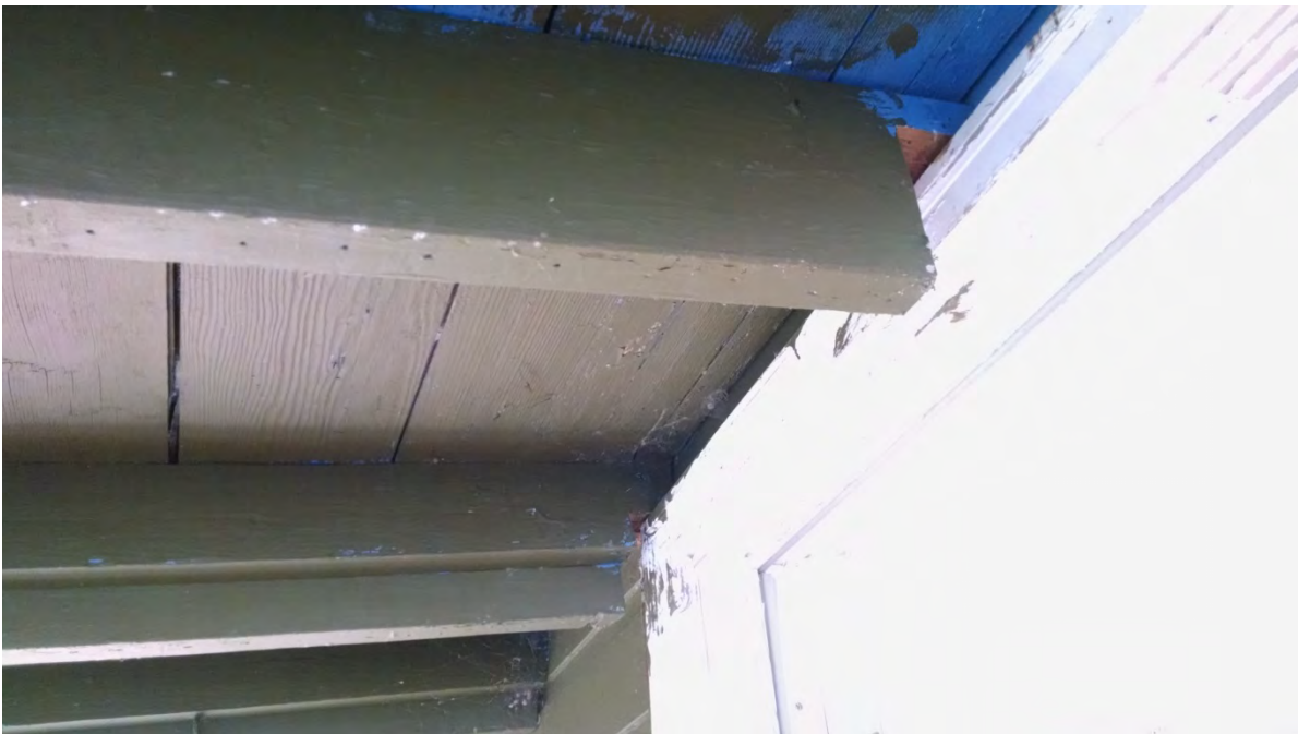
Notched rafters over doorway into caretaker's building
