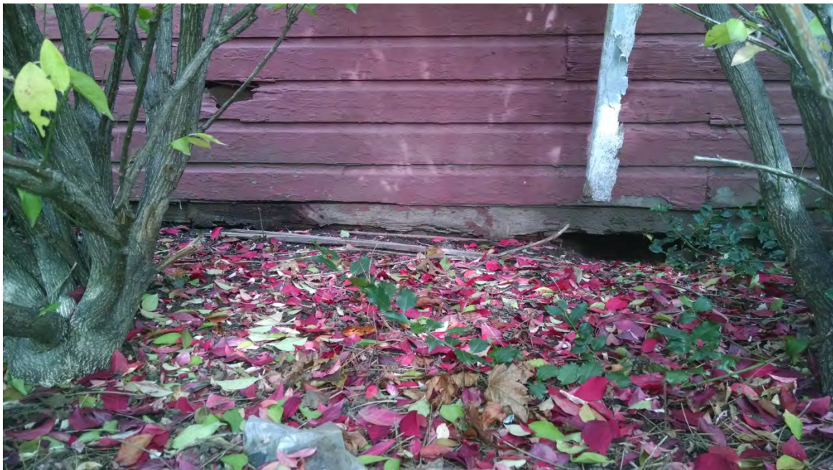
Siding in contact with ground
