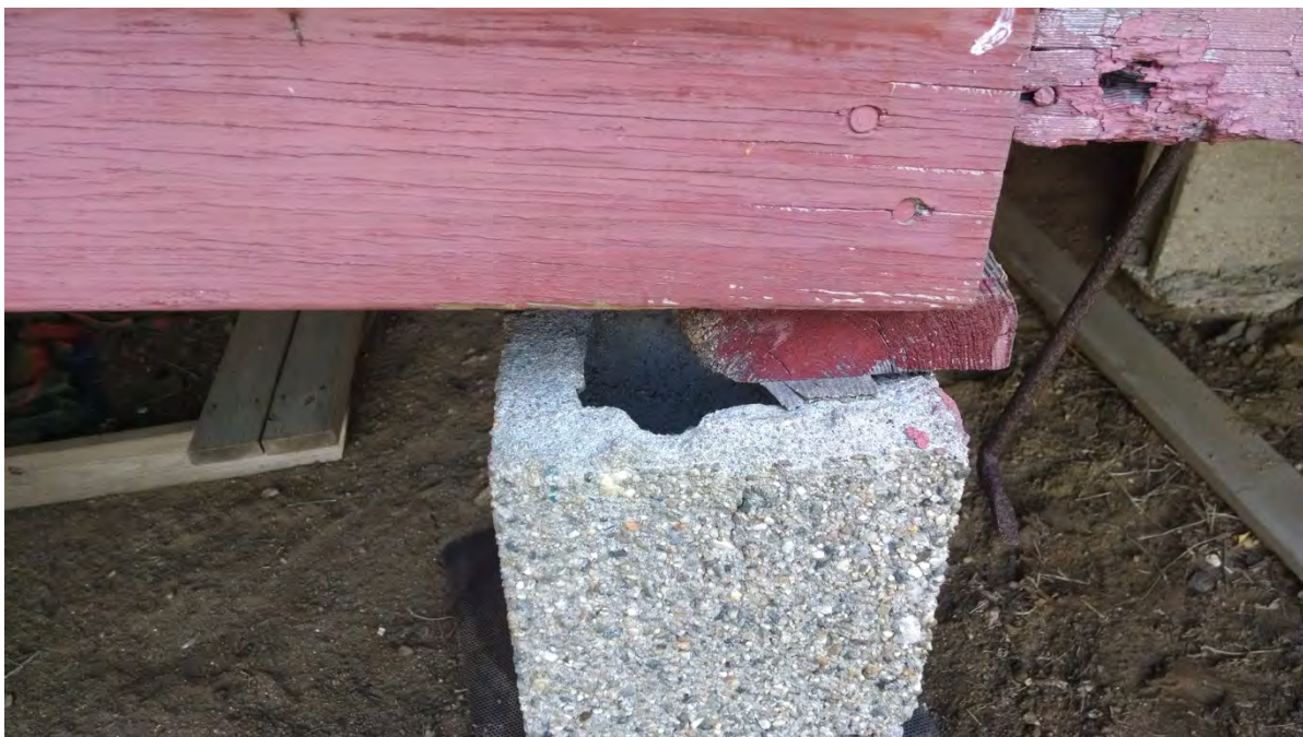
Typical unrestrained pier to beam connections
