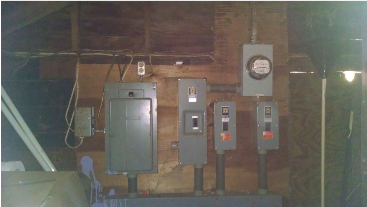
Primary electric service feeds Main, Boy's, Girl's and Caretakers buildings.
