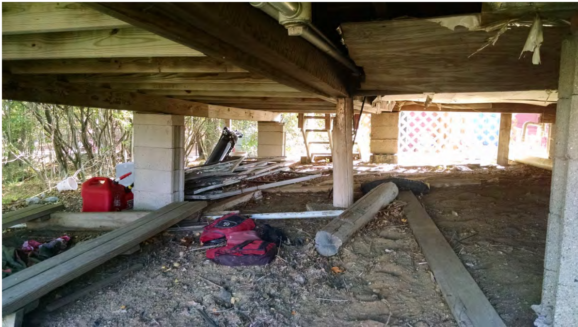
Typical pier construction
