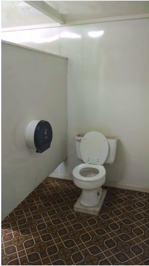
Non-compliant accessible toilet stall
