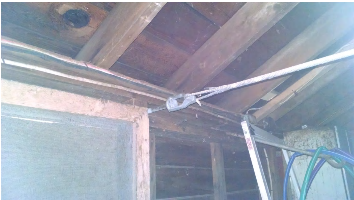
Steel cables added to prevent outward roof thrust.
