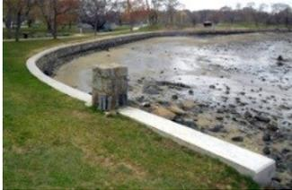
**Salem Willows Seawall** – In 2008 the Salem Willows seawall project was completed. This project repaired a crumbling 75 year old seawall that protects the edge of the existing park from the sea.
