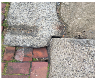
Figure 4a: Hole found at the perimeter of the building
