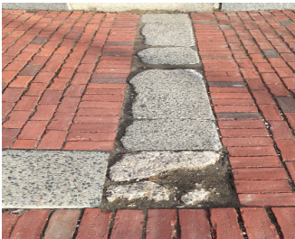
Figure 3: Granite paver in poor condition
