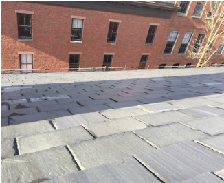
Figure 4: Snow guard at the roof perimeters
