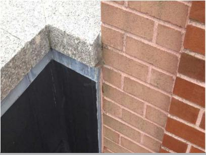
Lead coated copper through wall flashing, weep holes, termination LCC flashing, membrane flashing and stone ballast.
