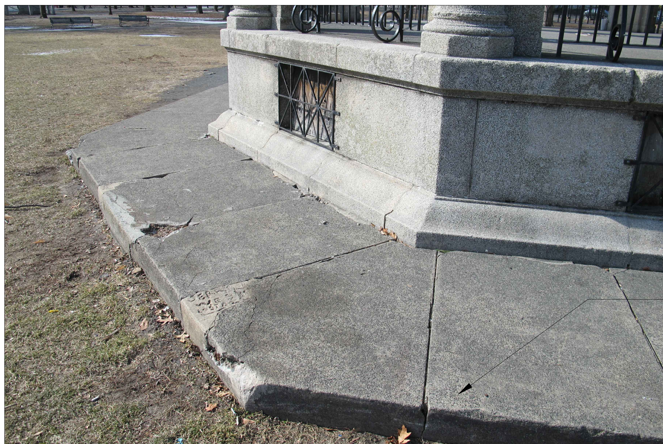
1 DETERIORATED PERIMETER CAST-IN-PLACE CONCRETE APRON
