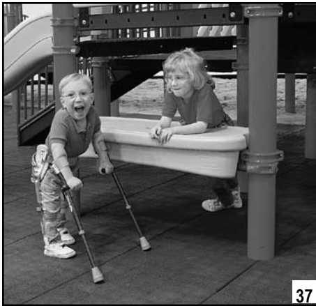
Rubber surfacing tiles facilitate access in this play area.
