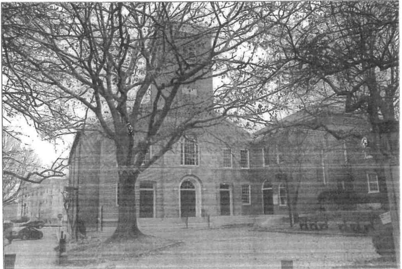
Photo 1 – Church façade (south) with Chapel addition
