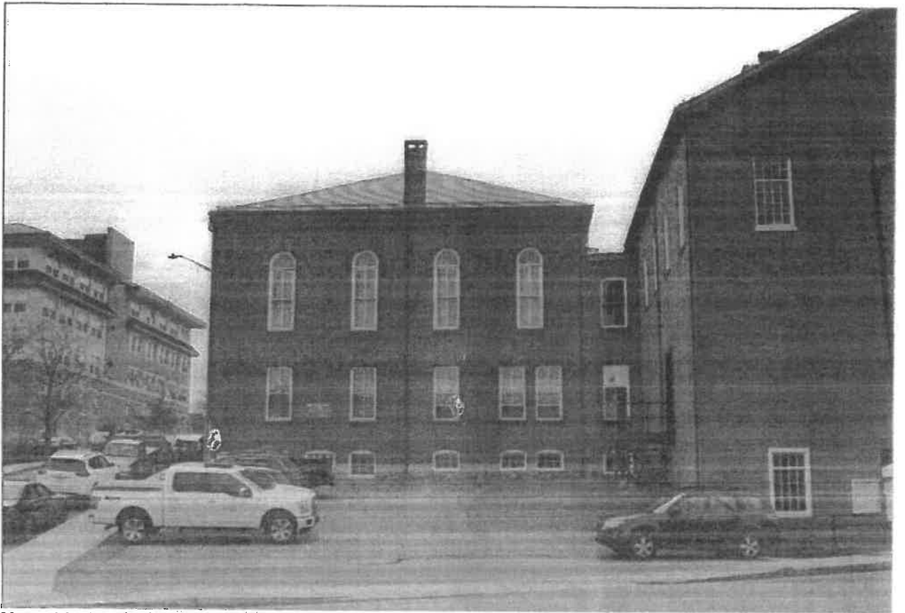
Photo 14 – North elevation of Chapel and ell
