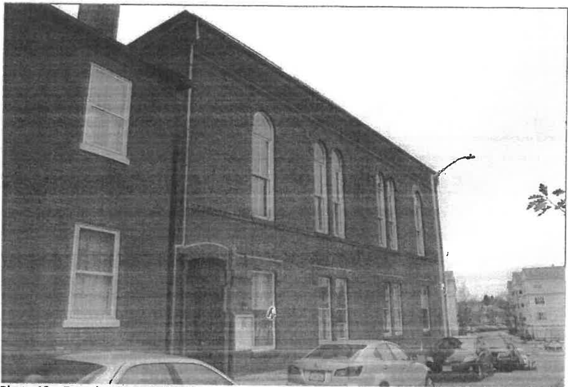
Photo 12 – East elevation of Chapel
