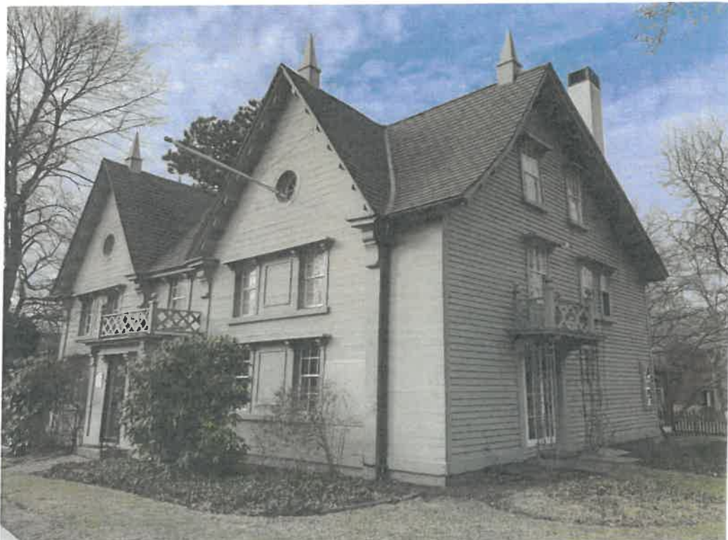
Photo #3: View of front (South) and East facades, Broad Street
