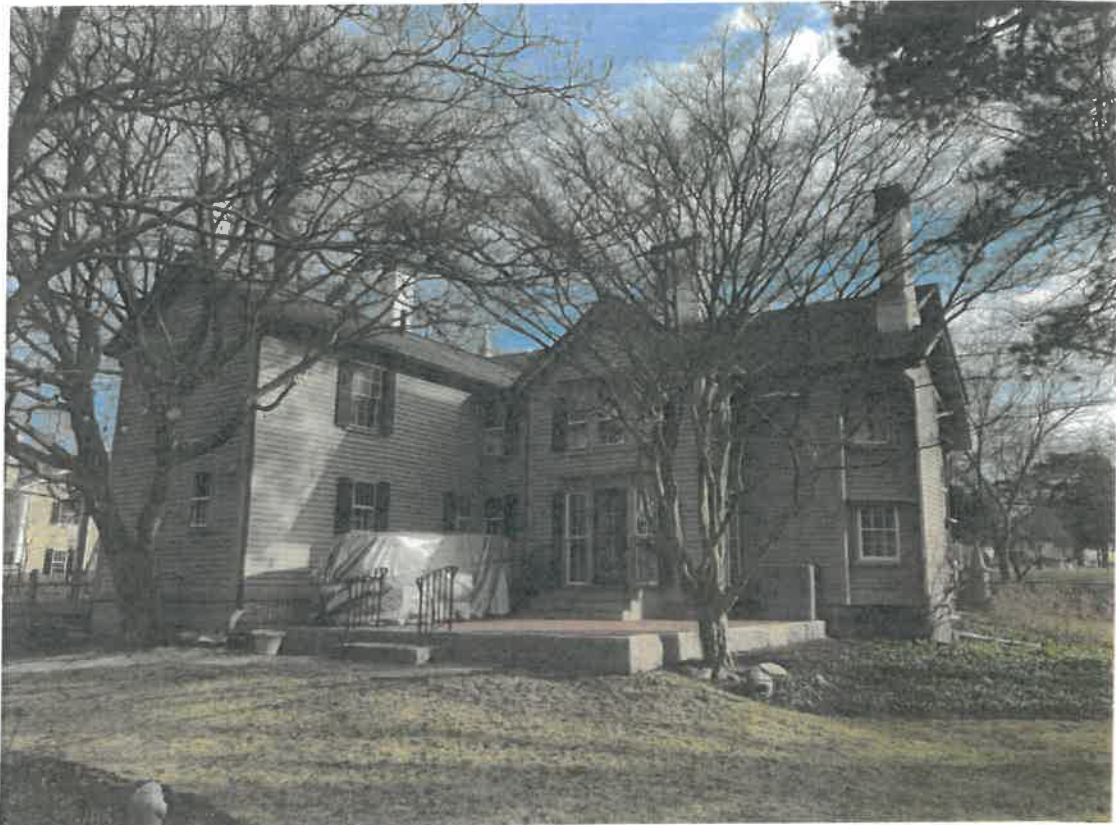
Photo #7: View of North elevation
