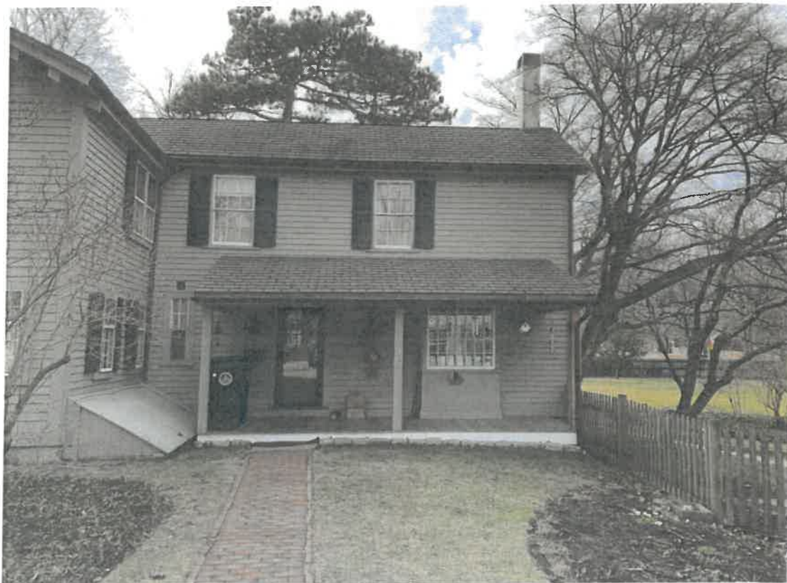
Photo #8: View of rear ell, East elevation
