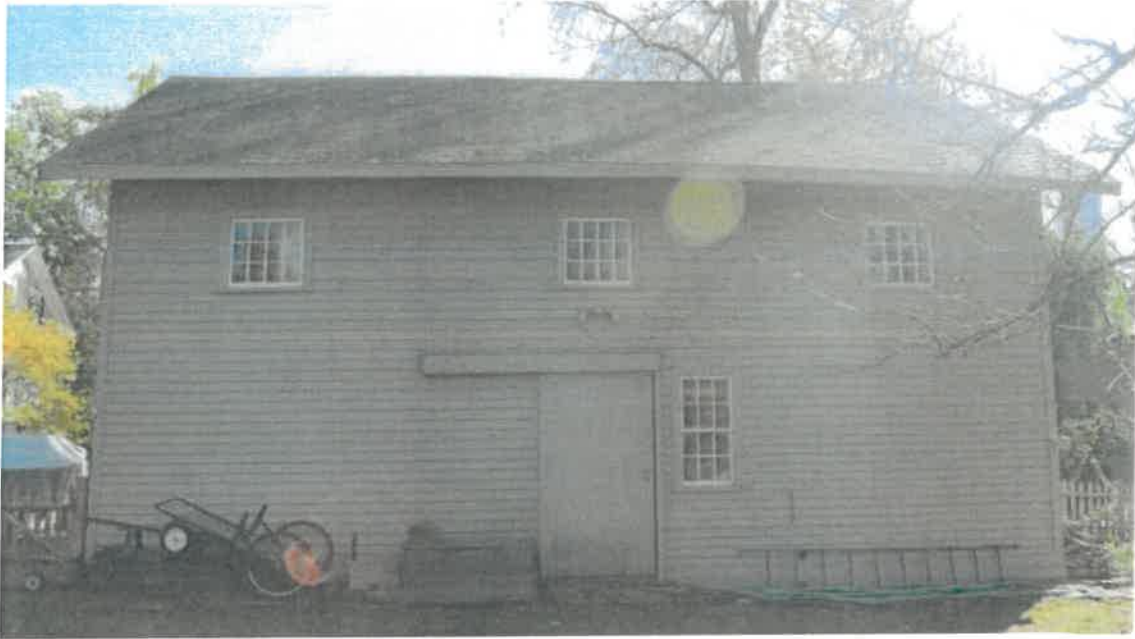
Photo #12: View of Barn, north façade Provided by Pickering Foundation, November, 2022
