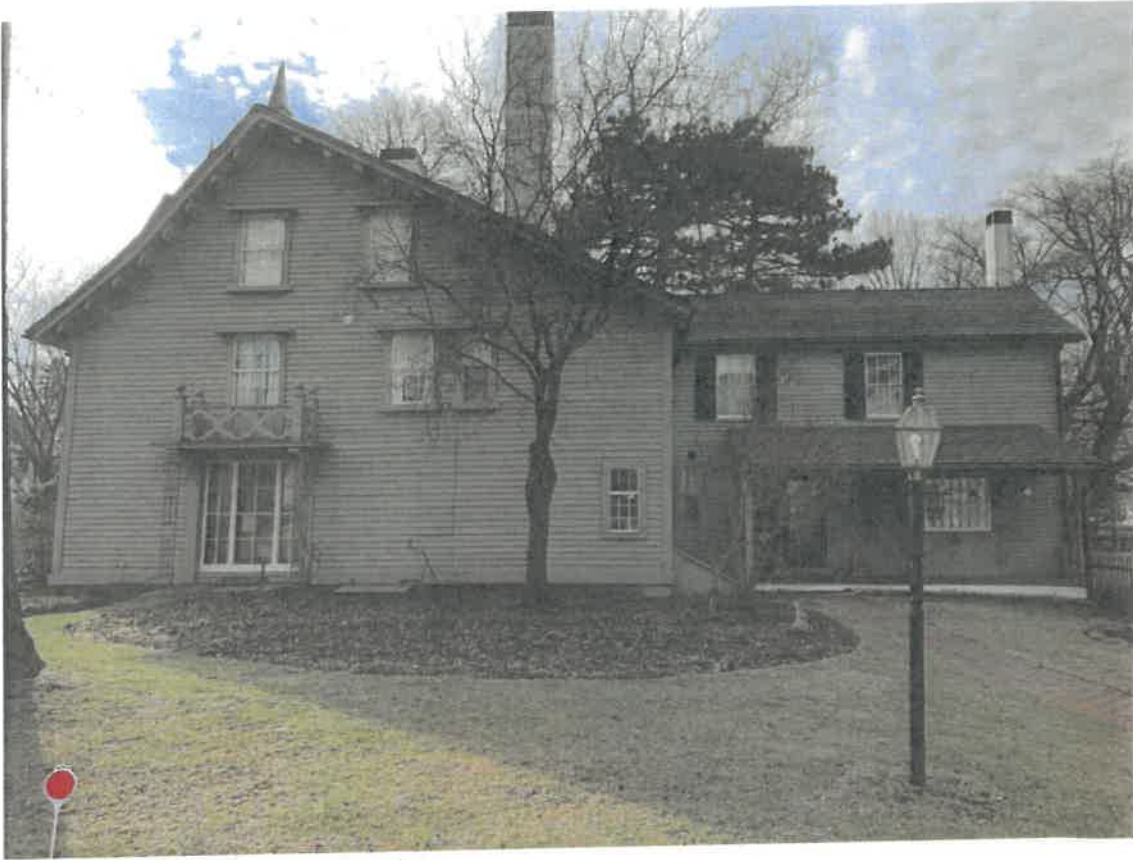
Photo #4: View of East elevation
