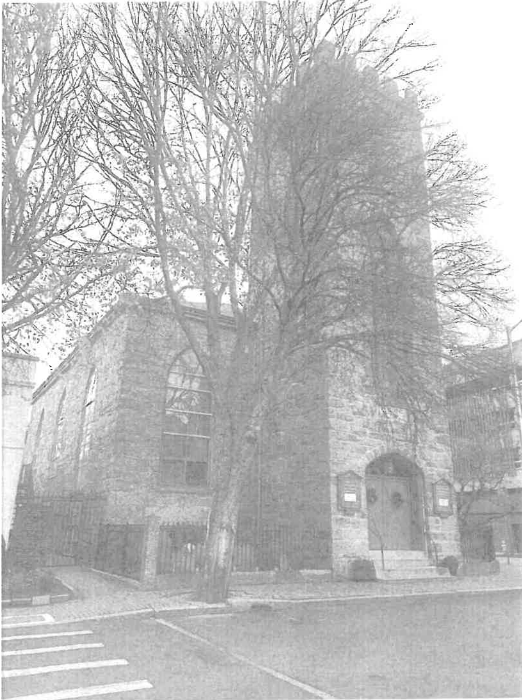
Photo 1 - Front facade (West and North elevations) December, 2022
