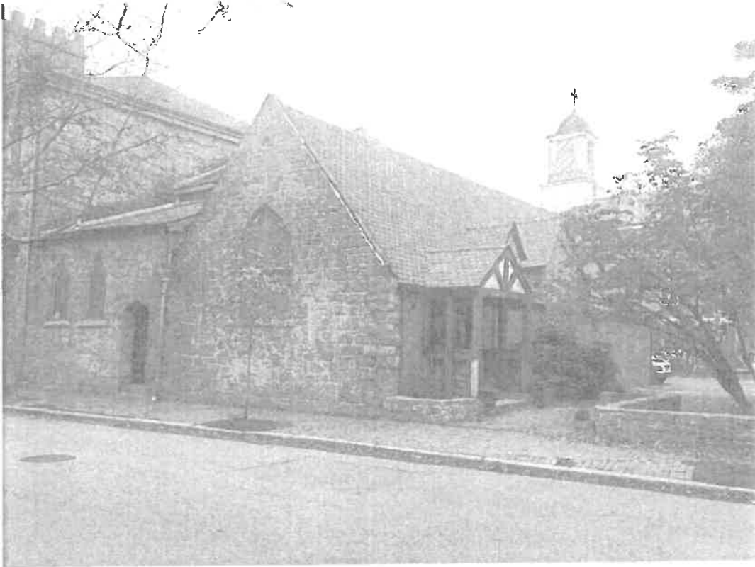
Photo 7- Chapel Addition (South and East elevations) - December, 2022
