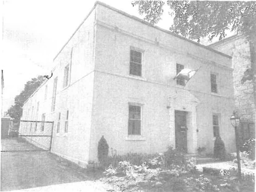
Photo 13 - Parish House (North & West Elevations) - May, 2023
