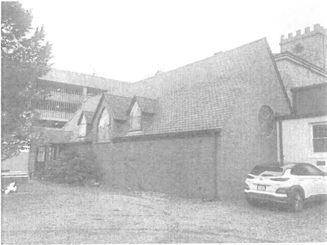
Photo 9- Chapel Addition (East and North elevations), connected to Parish House - December, 2022
