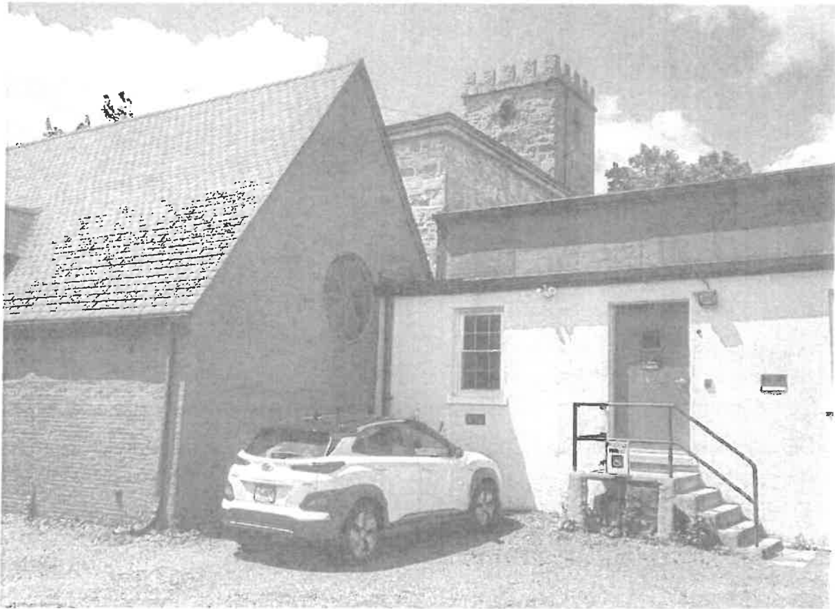
Photo 11- Chapel addition (North elevation) connection to Parish House rear (East elevation) - May, 2023
