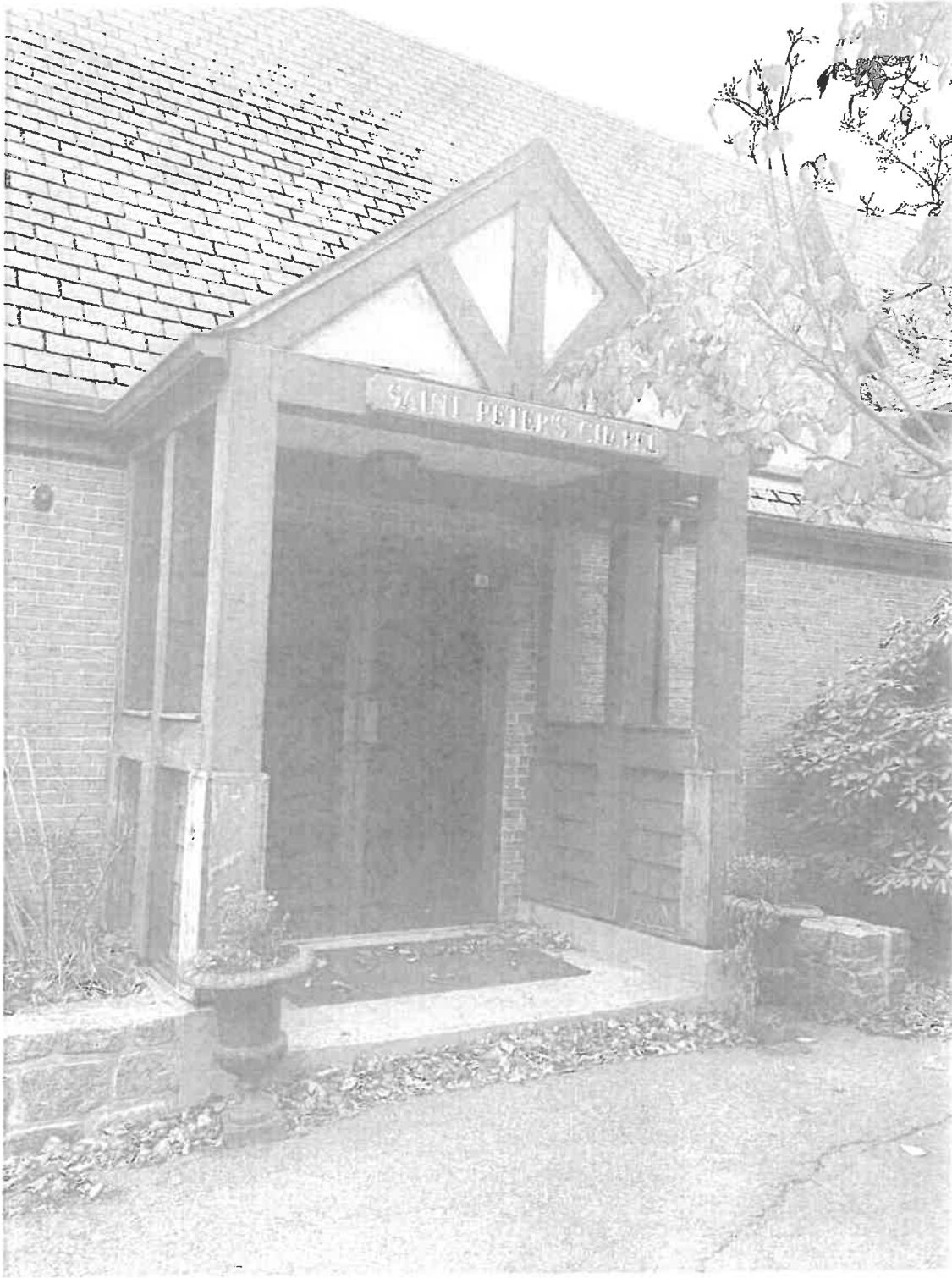
Photo 10- Chapel Addition Door (East elevation) - December, 2022
