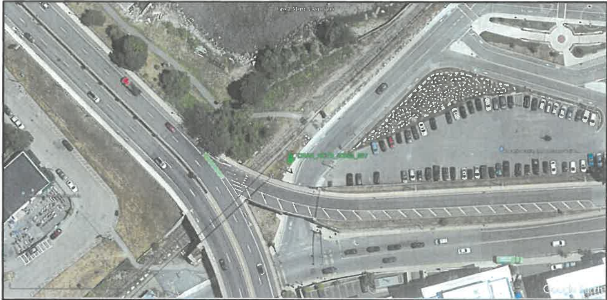
Figure 2: Utility Pole Within Salem, MA Proposed to Host An AT&T Mobility SC PWS Facility. (Picture courtesy Google Earth ©2023 and may not represent current conditions)
