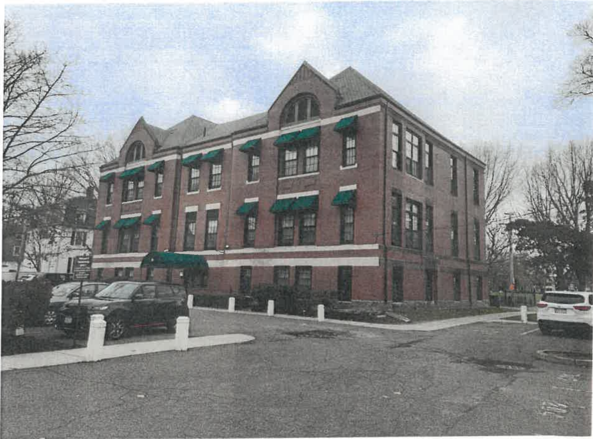
Photo 3- Rear (South elevation) December, 2022
