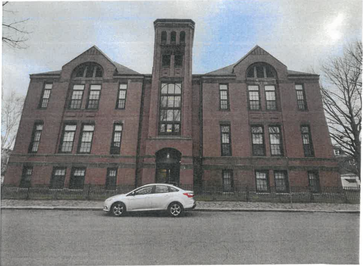
Photo 1- Front façade, South Washington Square (North elevation) December, 2022
