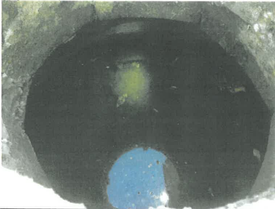
Figure 7 - View MH#3 and the submerged inlet pipe from CB#1 (photo taken 10/22/18).
