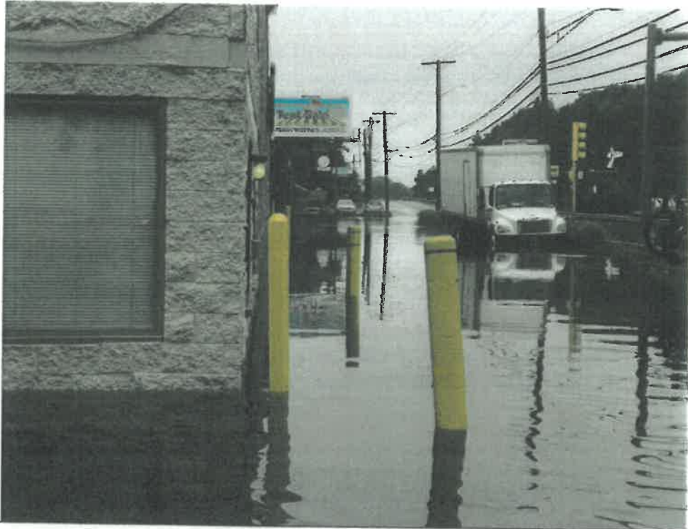
Figure 1 - View the Life Storage building (left) and Highland Avenue (Rt. 107) flooded.
