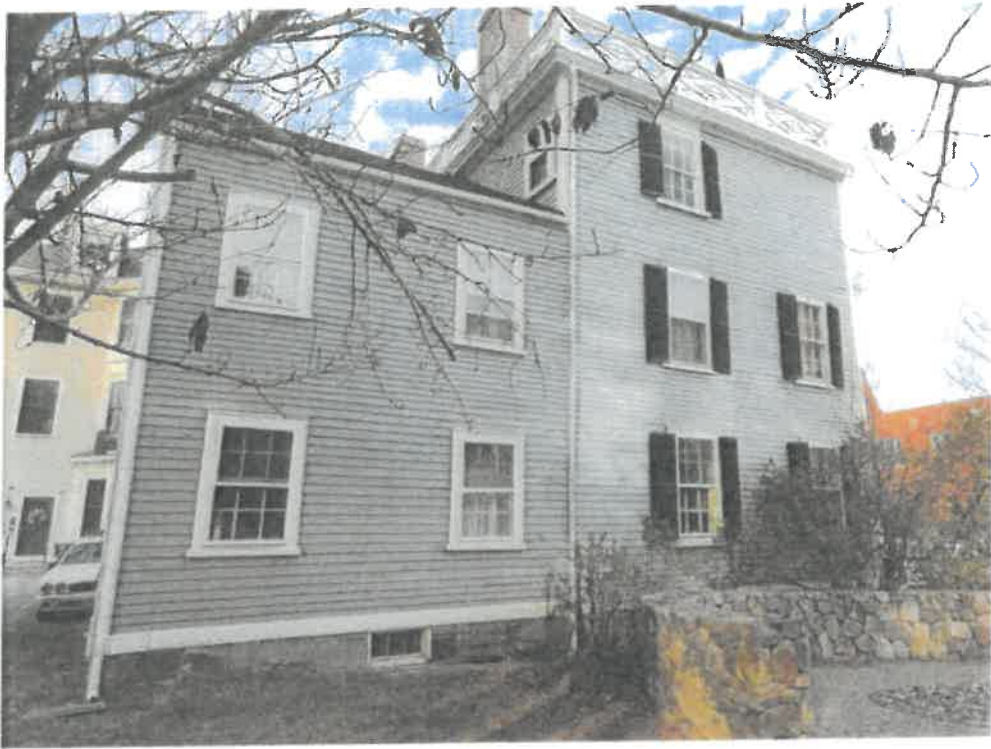
Photo 5 – Rear Addition, South elevation
