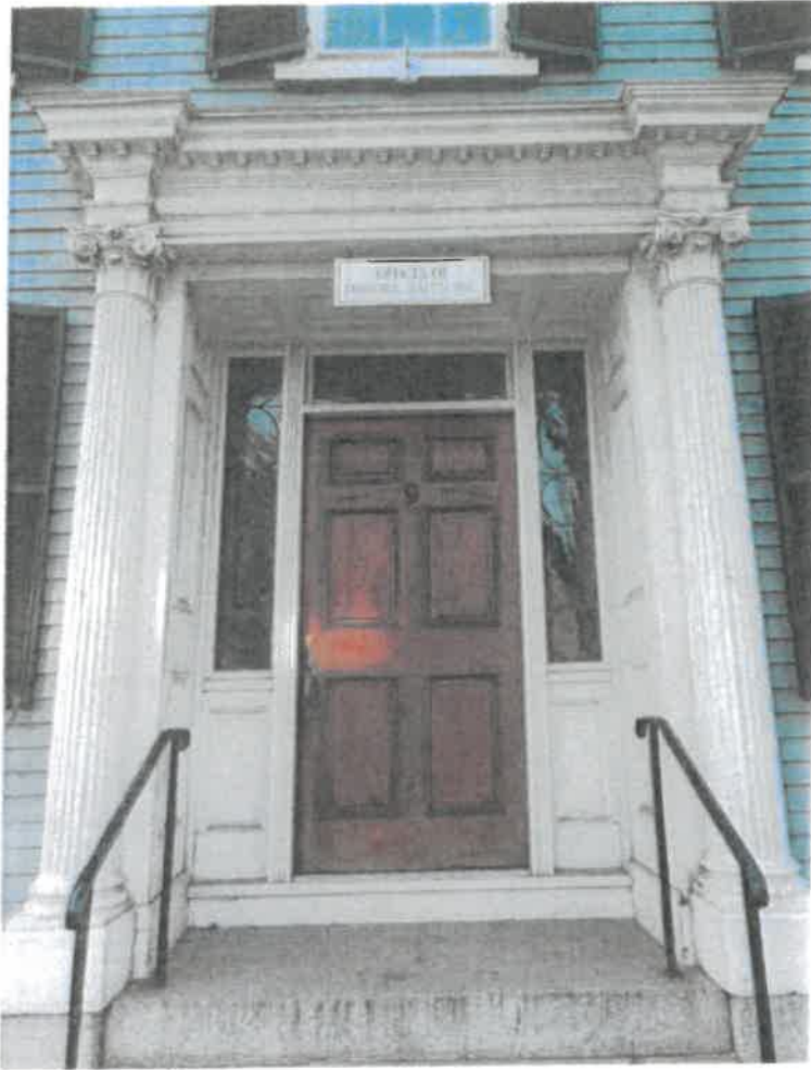
Photo 6 – Door Detail Main Façade (East Elevation)
