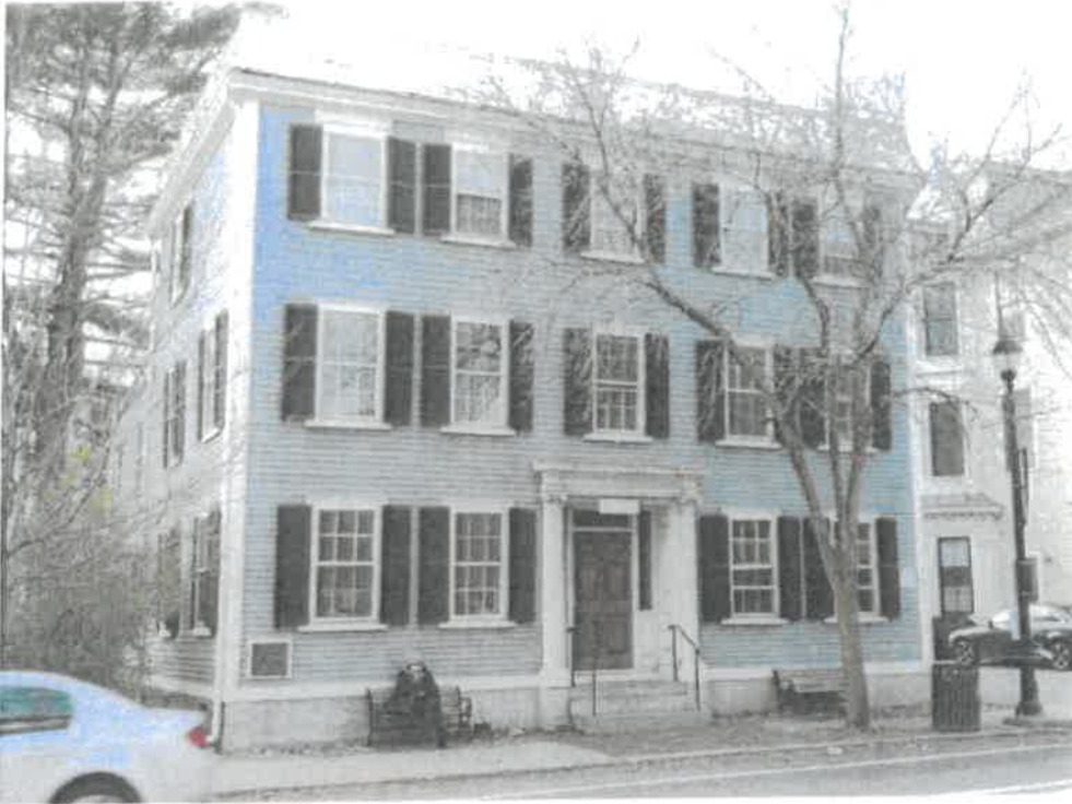
Photo 1 – Main Façade (East Elevation)
