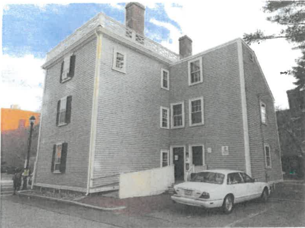
Photo 3 – Rear Addition, West elevation
