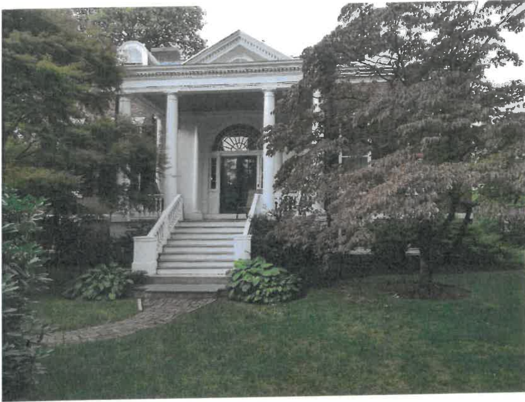
Photo 2 – Rear façade (South elevation)
