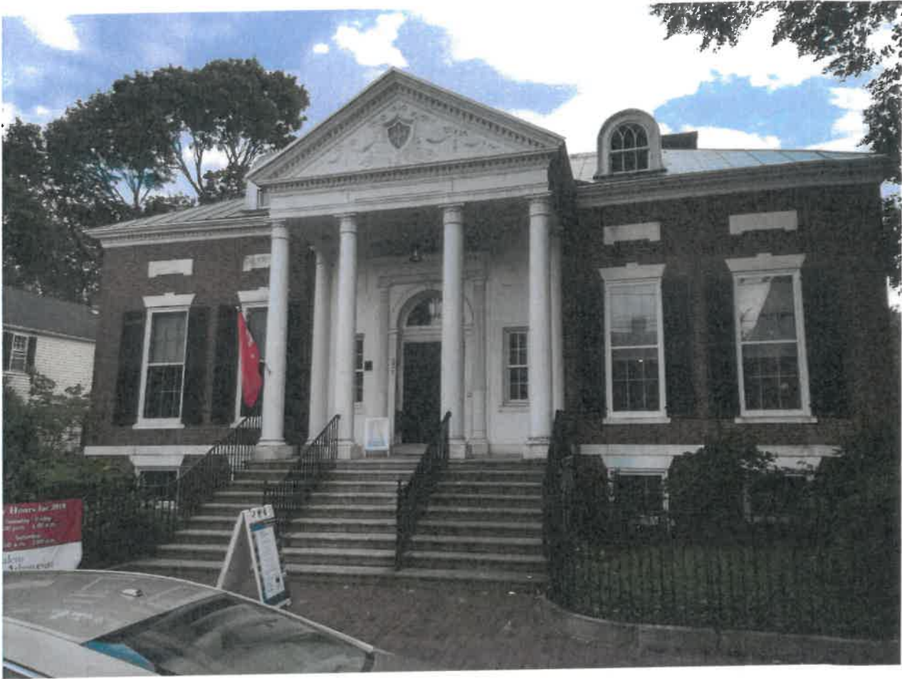
Photo 1 – Front façade (North elevation)
