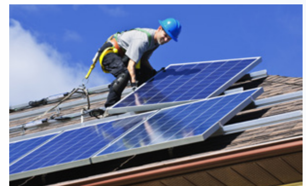
Installation of photovoltaic panels.
