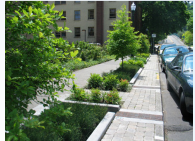
A green infrastructure containing a bioretention area.
