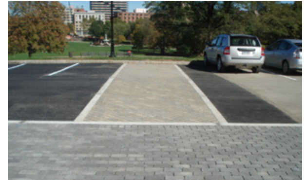
Permeable pavement and porous concrete sidewalks at the capital building in Harford CT.
