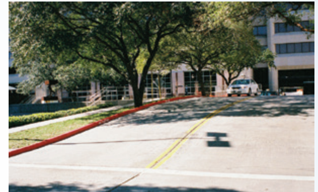
Ross Sterling Avenue was raised to protect the MSB to the level of the base flood.
