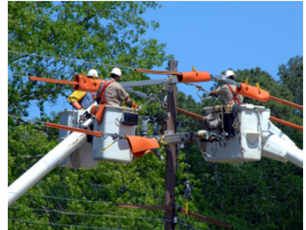
Electrical crew repairs damaged electrical distribution system after a storm.
