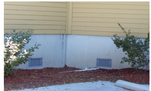
Non-residential structure retrofitted with flood openings.
