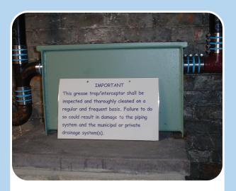
Grease traps like this one are installed between kitchen fixtures (like 3 bay sinks) and the building sewer, and collect grease. If not maintained, the grease laden wastewater bypasses the trap and goes out to the sewer. The grease eventually congeals and leads to sewer blockages.
