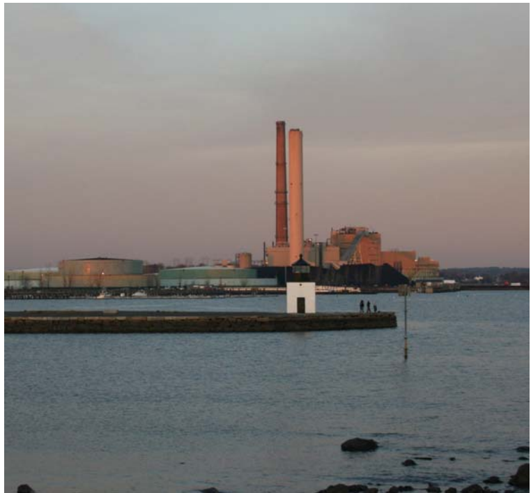
Derby Light and Salem Power Plant
