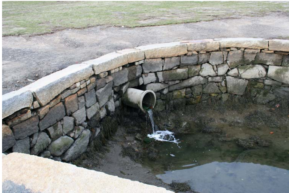
Outfall at End of Derby Wharf
