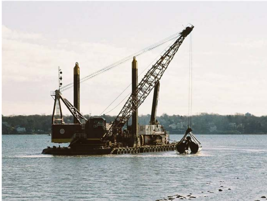
Army Corps of Engineers Dredging Project (2007)
