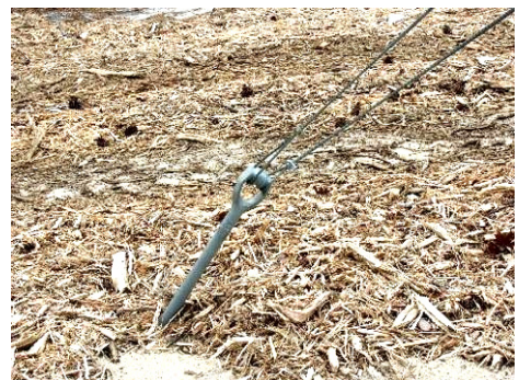
An anchor, installed, with 2 guy wires attached
